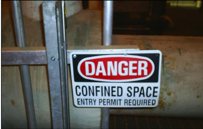
Figure 39: This is displayed as a confined space. However, many confined spaces are not so well defined. In particular, maintenance of a vessel, a cold box or a not well-ventilated space which requires entry would need oxygen monitoring and a special confined space entry permit
